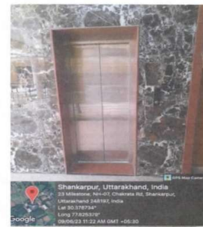
Availability of Lift Facility for All
