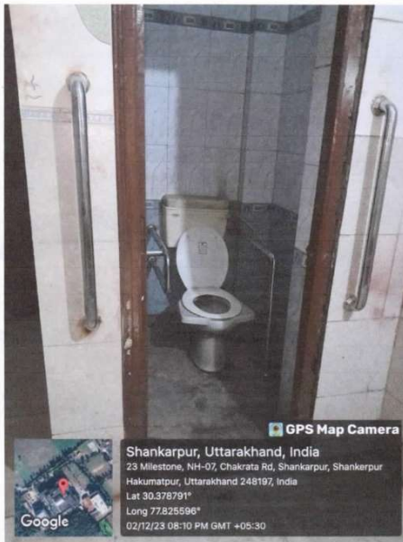
Disabled Friendly Wash Room
