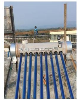
Fig.3 Evacuated tube solar water heater [19]
